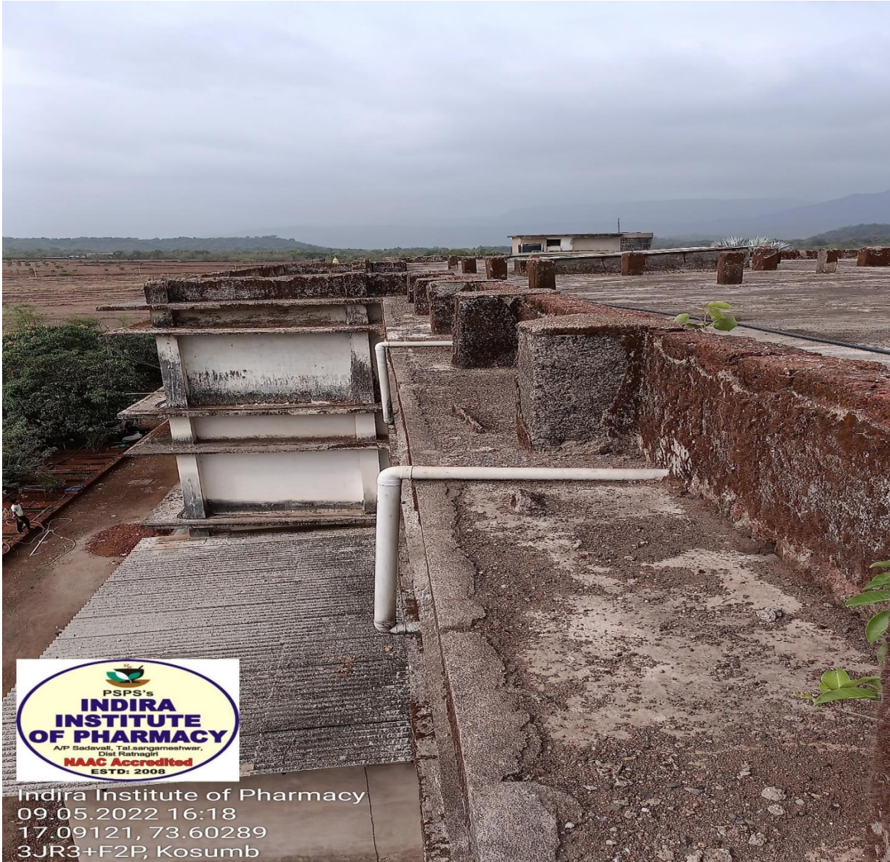
Rain Water Harvesting System
